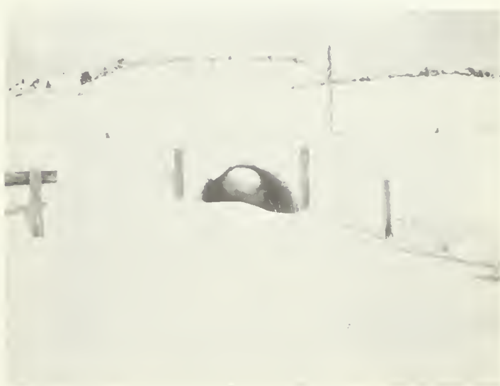
SOUTH ENTRANCE: drifting severe.
